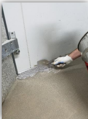
16. Pre-primed substrate and slightly broadcasted
