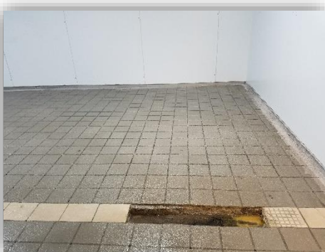
10. Holes need to be filled with mortar
