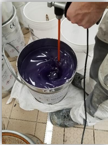
7. Mixing Plastifloor®112 with Hardener 50W
