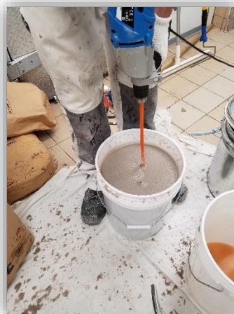
11. Mix Plastifloor® 510 with mix C2 and Hardener
