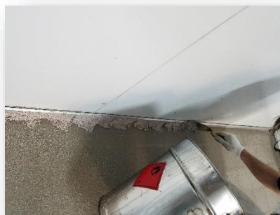
17. Use spatula to equally spread the mixture
