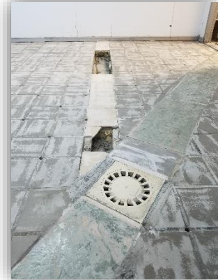
3. Substrate ready for priming
