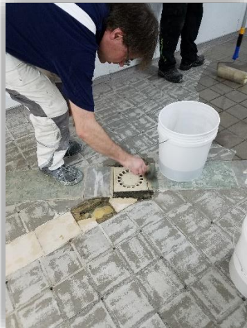
8. Priming the details with brush first
